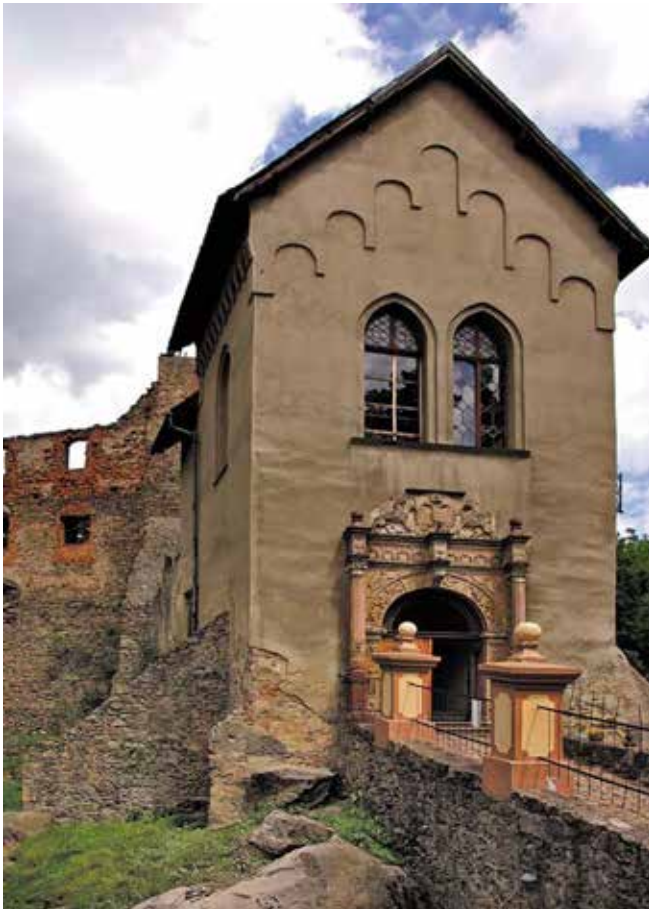
Castle Grondo: the finely carved stone of the door surround contrasts with the ruinous state of adjacent walls. Photo Agnieszka Kaluzny
